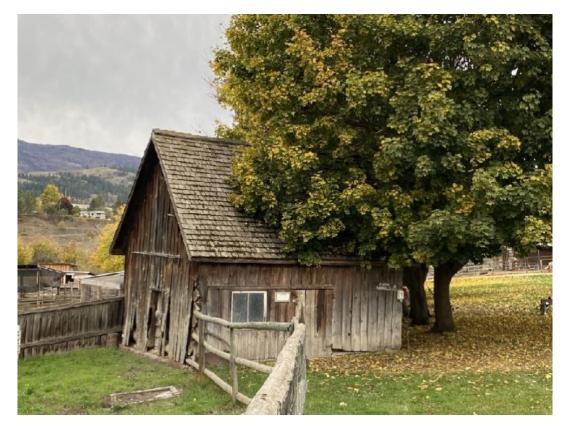
Pioneer Log Cabin - later the Chicken House ca. 1867. The log structure is visible beneath the board and batten cladding.
