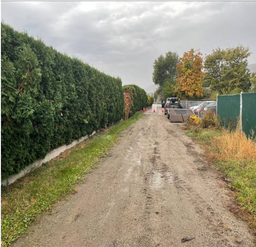
Cedar row being removed
