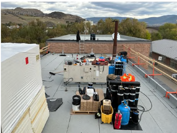
VWRC two completed roof sections.
