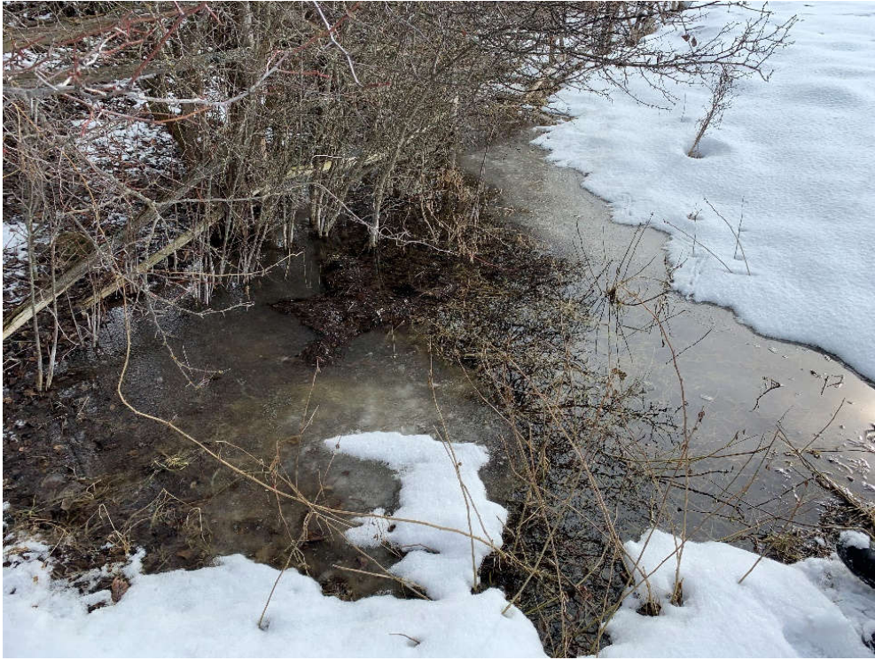
Photograph 5. View of pooling water on the Property (February 25, 2021).
