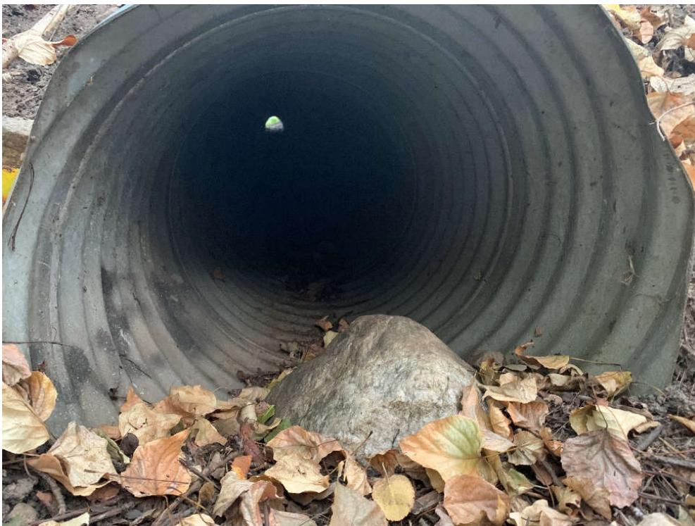
Photograph 18. Downstream view of the culvert inlet (September 28, 2022).
