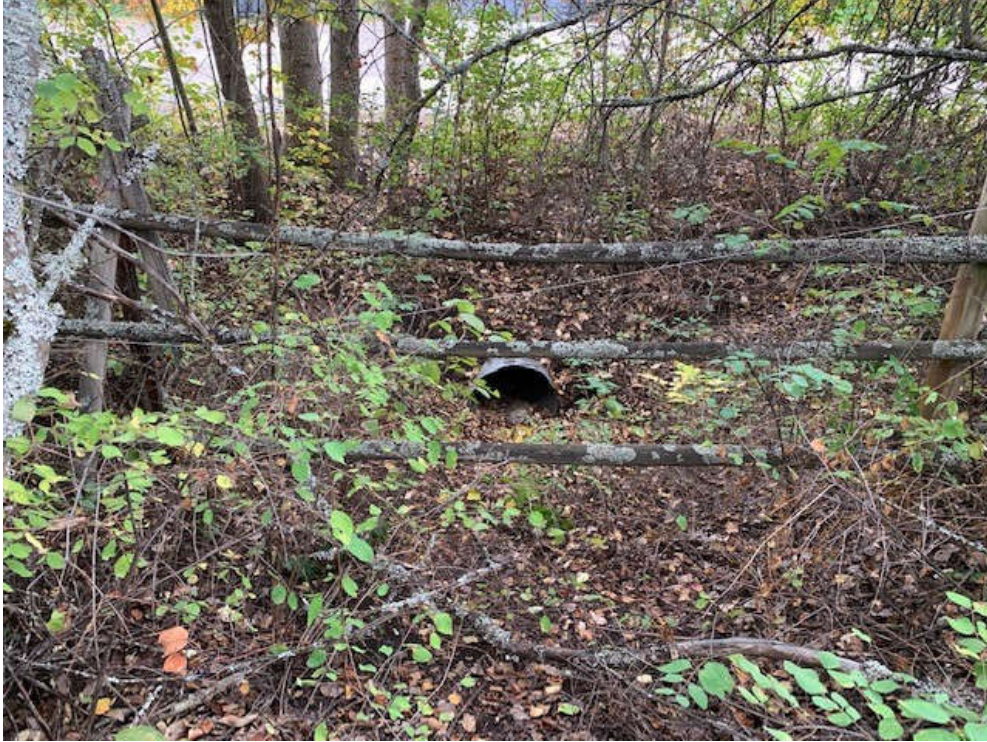
Photograph 17. Downslope view of the culvert inlet at Herbert Road (September 21, 2022).
