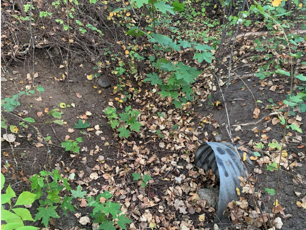
Photograph 19. View of the culvert inlet at Herbert Road (September 28, 2022).
