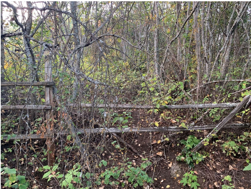
Photograph 20. View upslope of densely vegetated area upslope of culvert inlet (September 28, 2022).
