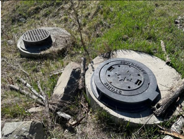
Photo 9: Existing manholes near middle west area of the Site
