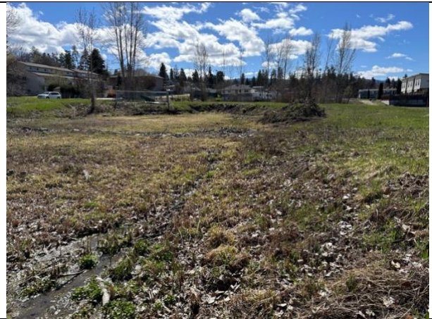
Photo 4: View of existing excavation at NW area of the Site looking south
