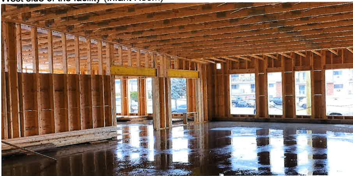
View looking from entry of 3-5 room towards adjoining 3-5 room.
