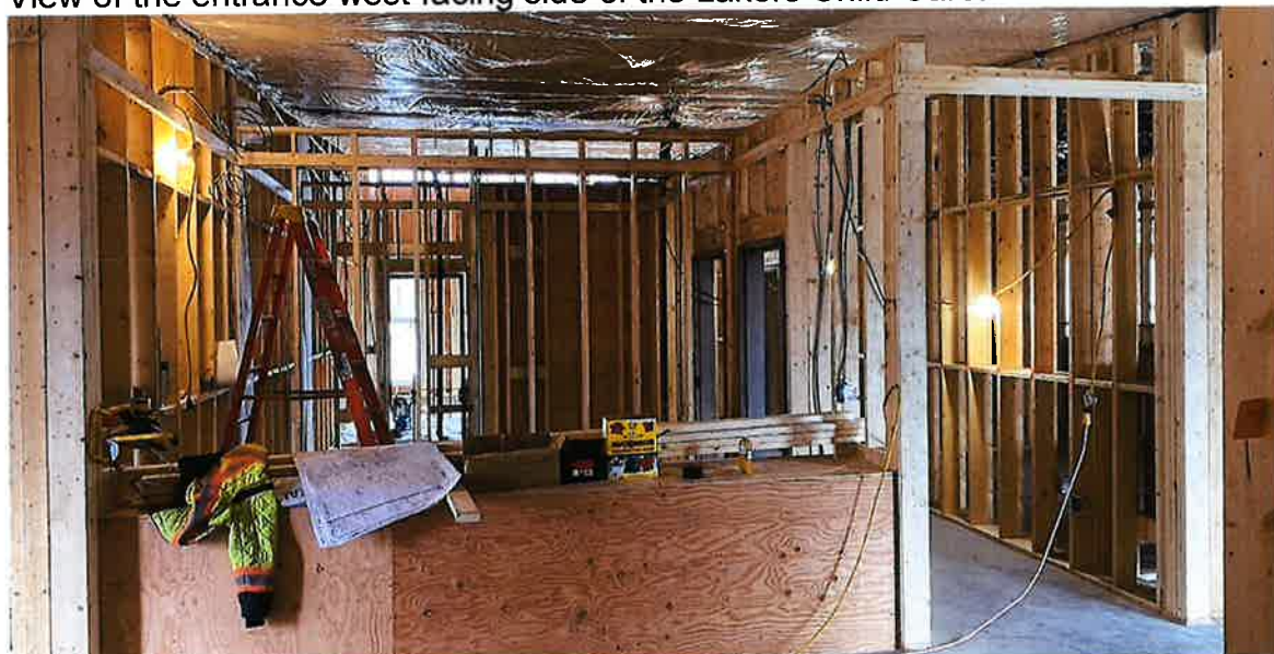
The entry way main reception desk.
