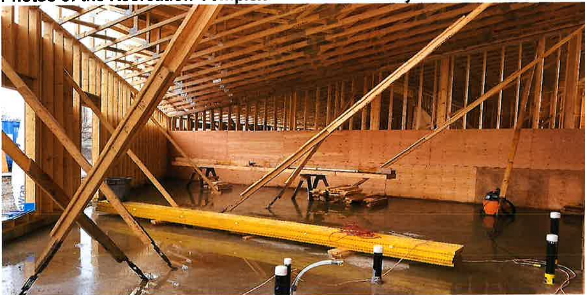
West side of the facility (Infant Room)
