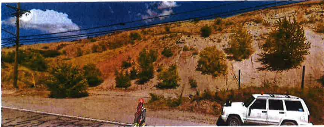
Figure 3: Street view at southeast corner of site, on Kalamalka Lake Road
