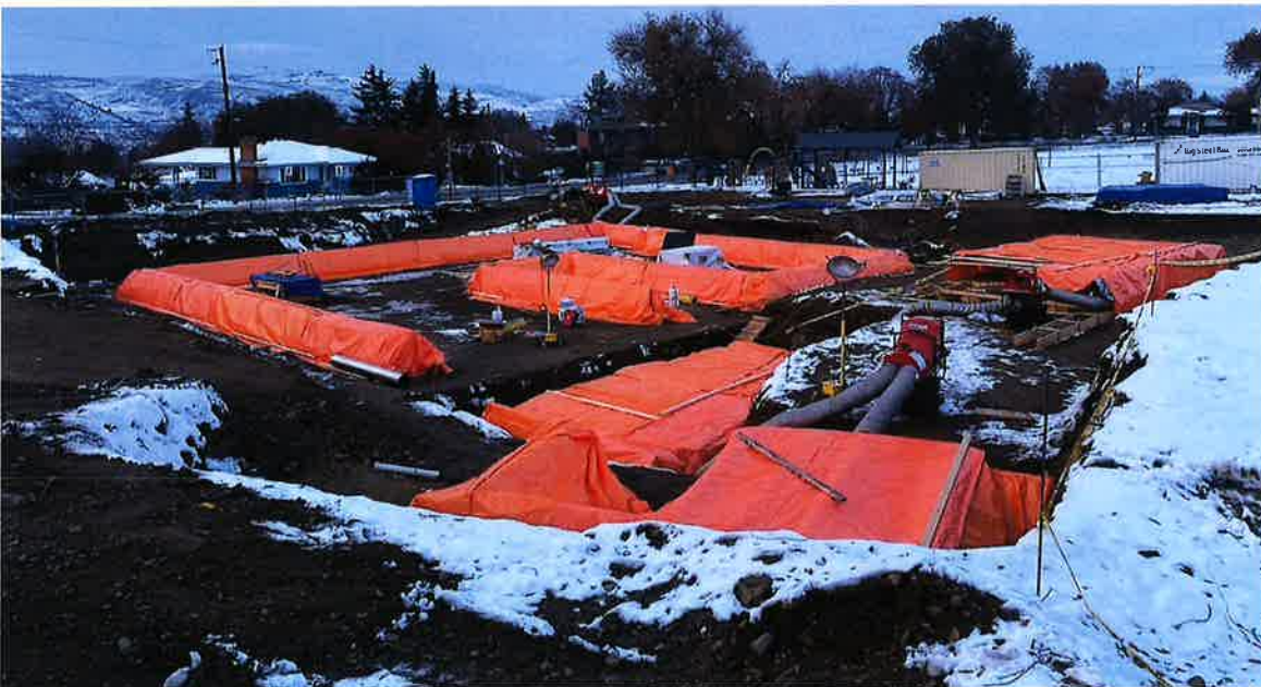
Heating forms for concrete footings
