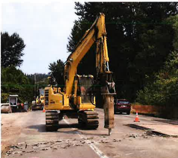
Excavator with boom attachment
