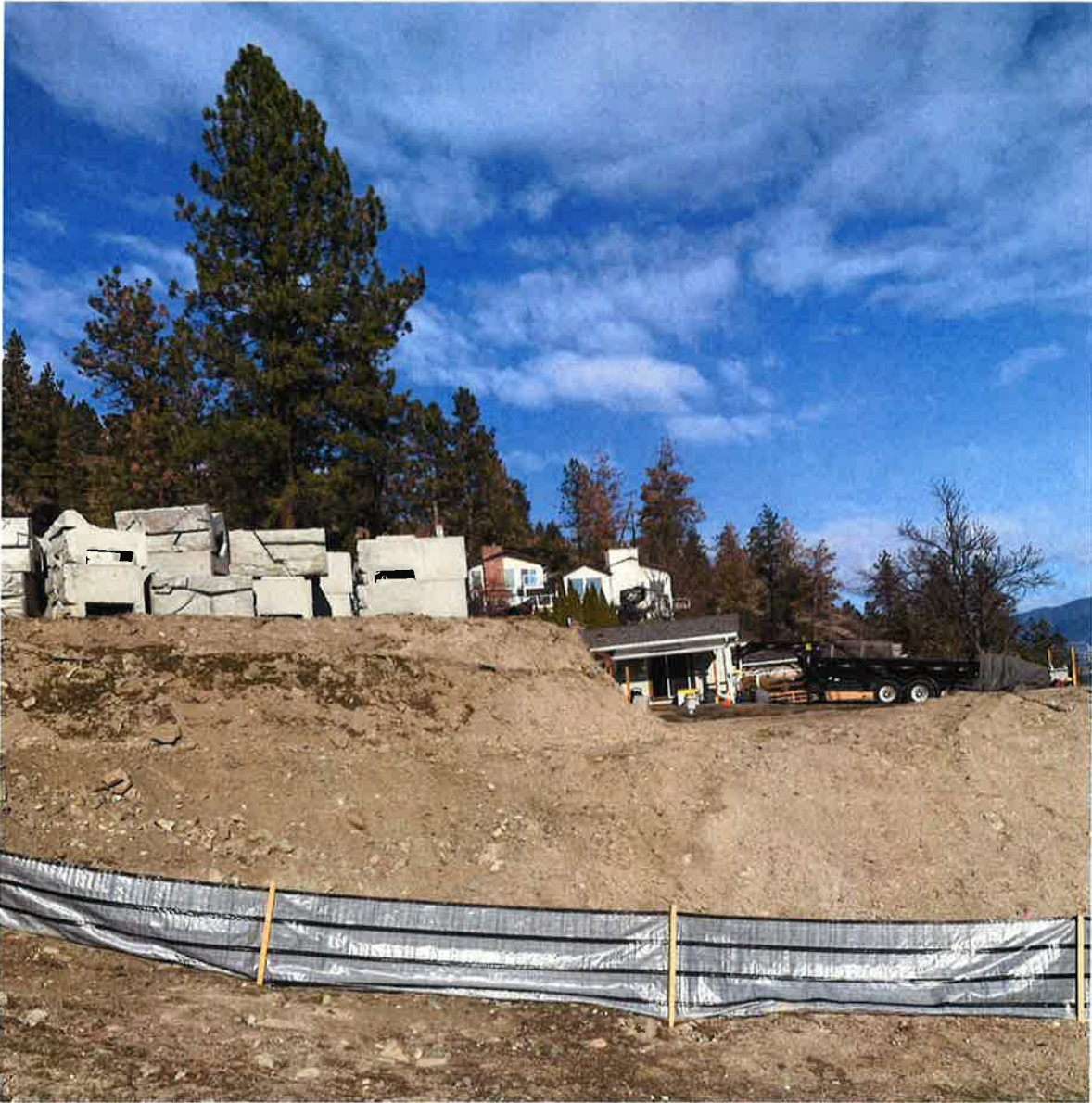
Photo 1: Verti-blocks, site fill and grading and silt fencing (approx. location of retaining wall)
