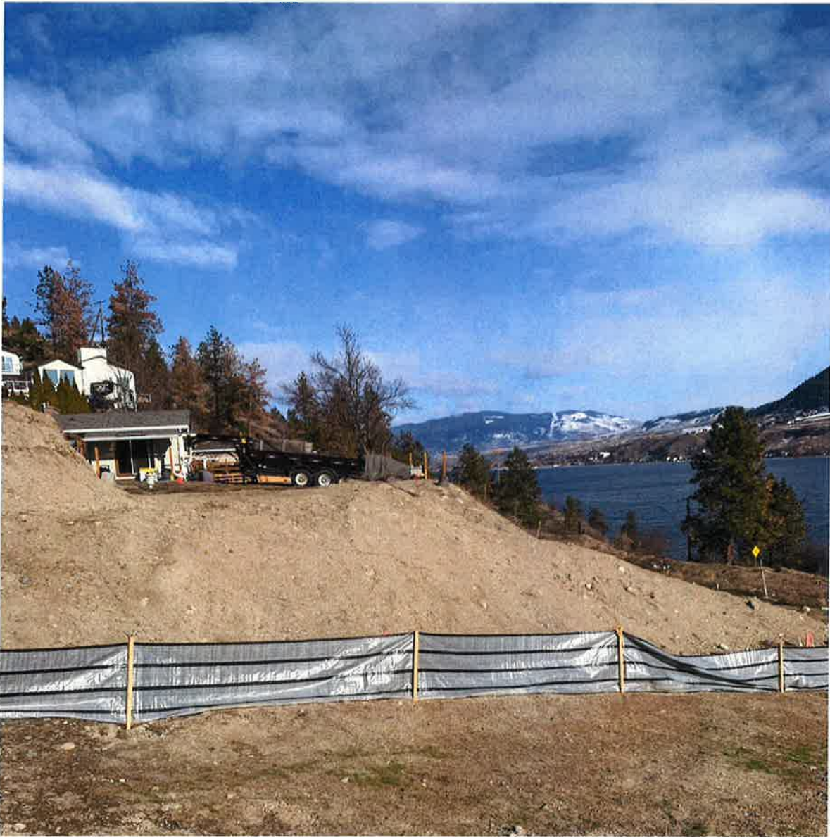
Photo 2: Site fill and grading
