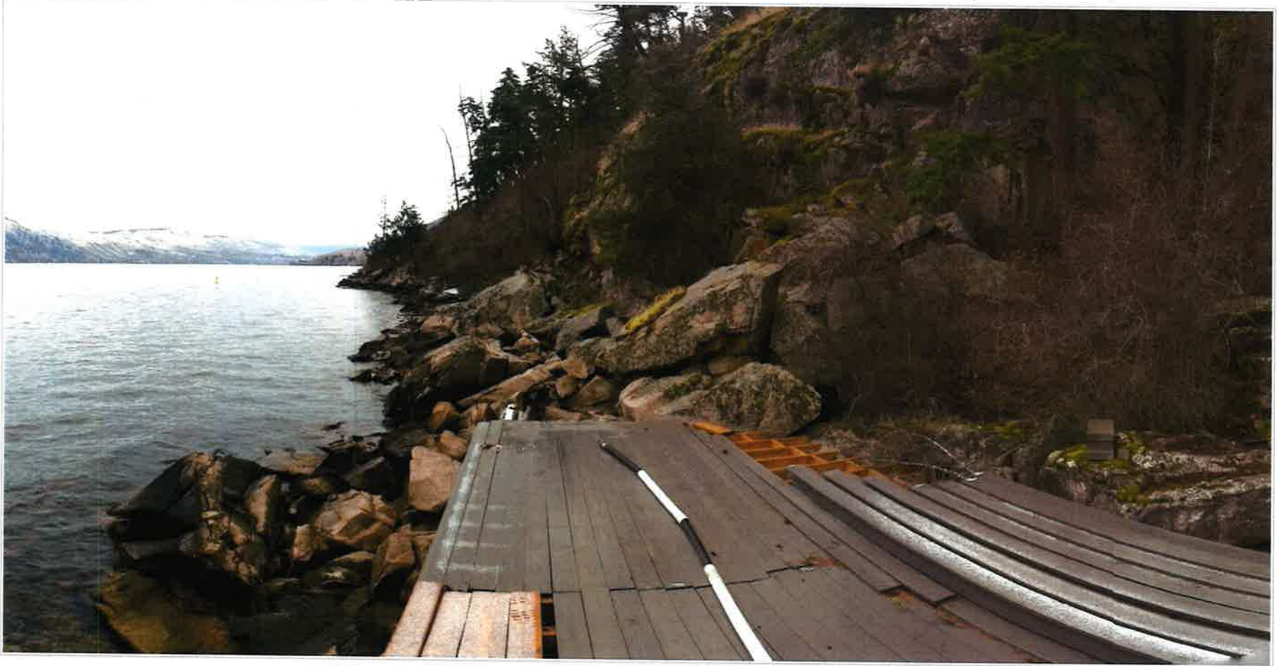
Photo 1. Foreshore, HWM / SB, SPEA vegetation, and existing deck to be removed (from proposed dock area - looking NE) – Dec. 14, 2020.
