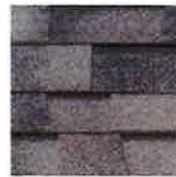
Roof Colour: Grey Asphalt Shingles
